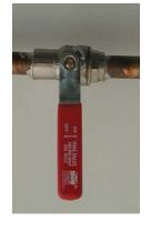
Photo 2b: Ball valve: closed position
